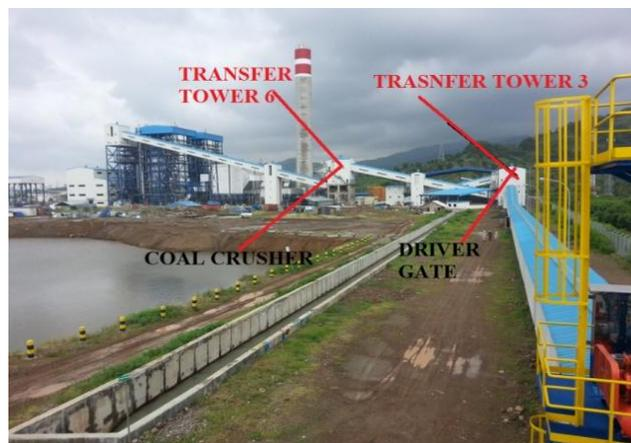
Gambar 3. Tata letak proses coal handling
